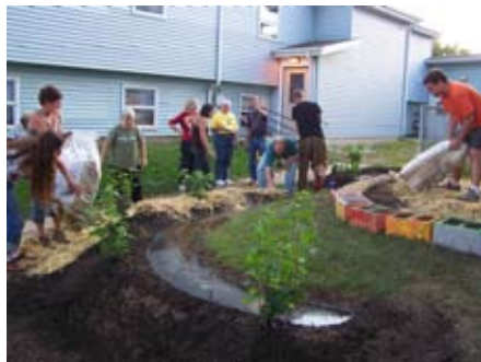
Class members built a swale to absorb rainwater from the building’s roof.
