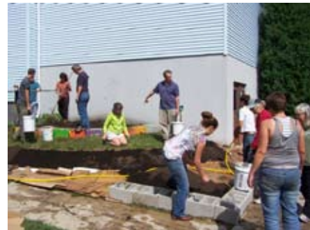
Cinderblocks were placed to serve as planters and a retaining wall.
